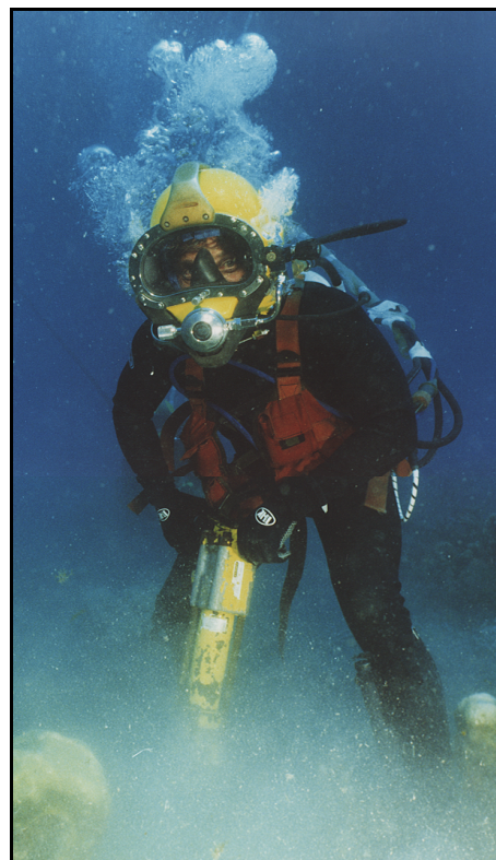
Figure 6-4. Underwater Construction Diving.
